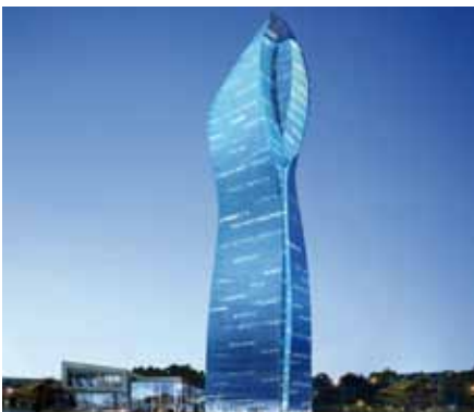
TUNED MASS DAMPERS
