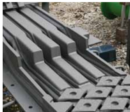
Guard rail of a low-noise expansion joint
