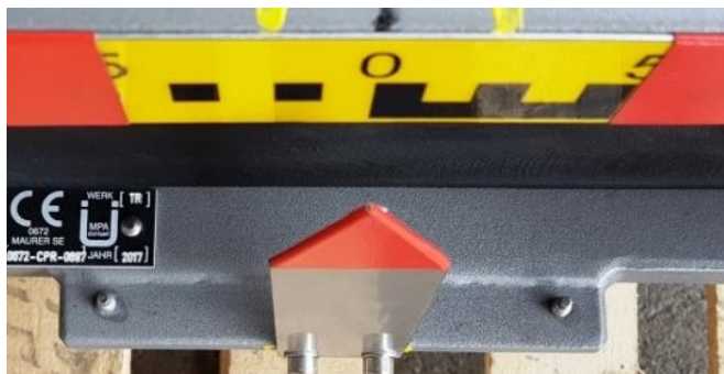
Figure 6: Two-point measuring plane integrated in anchor plate, top view of elastomer bearing
