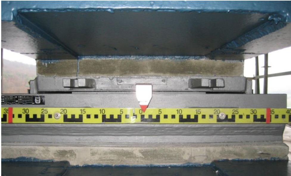
Figure 13: Grouting to steel substructure, grouting to steel superstructure
