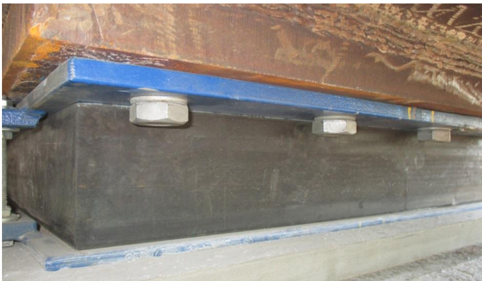
Figure 14: Grouting to the concrete substructure, bolted connection to the steel superstructure
