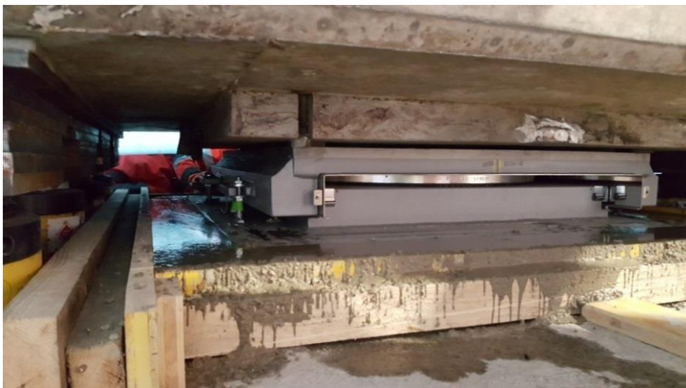
Figure 12: Grouting to the concrete substructure, welding to the steel superstructure
