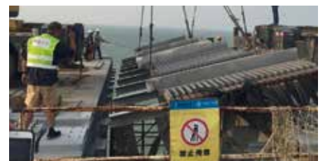
Inserting MAURER Sliding Lamella Joints into the structure
