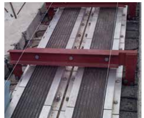
Installation of MAURER Double Mat Joints
