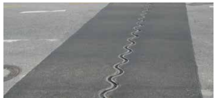
MAURER Low-Noise Single Seal Joint
