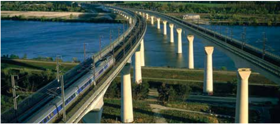
TGV railroad section near Avignon / France
