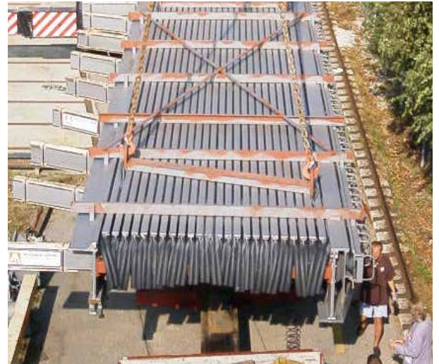
Joint with Fuse Box System type IV
