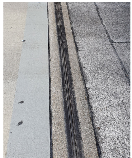
Elbepark Dresden: Compact expansion joint K30-B and D1-B with Betoflex®-anchorage for a car park
