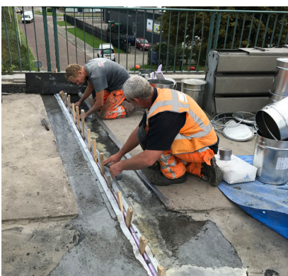
Fixing the gap width
