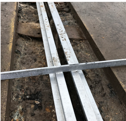
Aligning of the expansion joint
