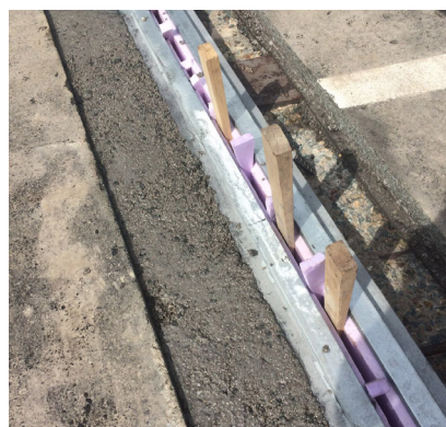
Header grouted on one side
