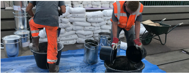
Mixing of Betoflex® on site
