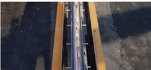
Compact Expansion Joint with Betoflex®-anchorage as longitudinal joint between two superstructures
