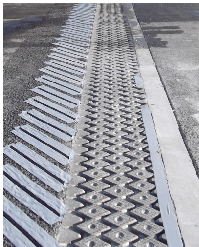
Expansion joint XD4 with stiffening ribs and Betoflex® header
