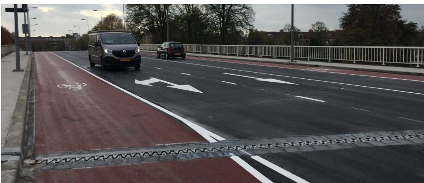
XC1-B joint installation examples
