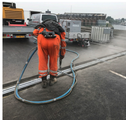
Abrasive blasting of the connection surfaces
