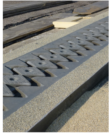
Expansion joint XD2 with transition Betoflex® header
