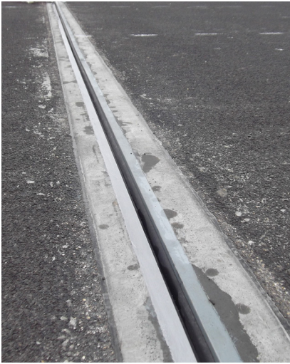
Viaduct Großenmoor: 8 expansion joints D1-B (125 m)
