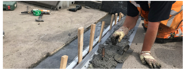
Installation of Betoflex®
