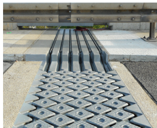
Transition beam at a multi-seal modular expansion joint
