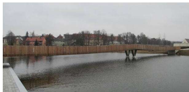
Fig. 28 – Footbridge for horticultural show in Tirschenreuth, Germany
