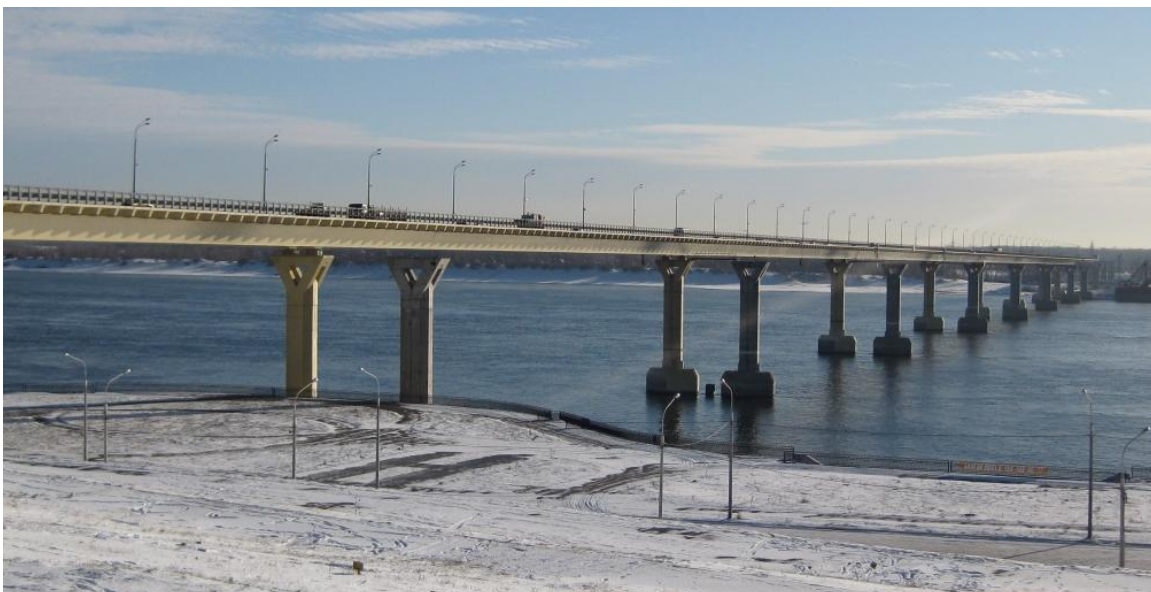
Fig. 22 – Volgograd Bridge, Russia
