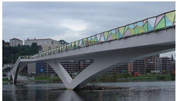
Fig. 27 – Coimbra Bridge, Coimbra, Portugal
