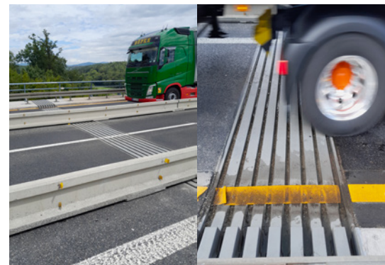
The installed joint under traffic.
