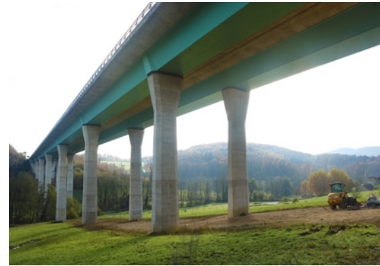
The Dultenaugraben Bridge between Lörrach and Rheinfelden.
