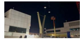
Installation of the SIP®-Bearings on top of the Y-columns. Work performed at night as the airport is being renovated while continuing to operate. *Photo: W&W* | AFCO Steel
