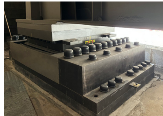
The fully installed bearing.
