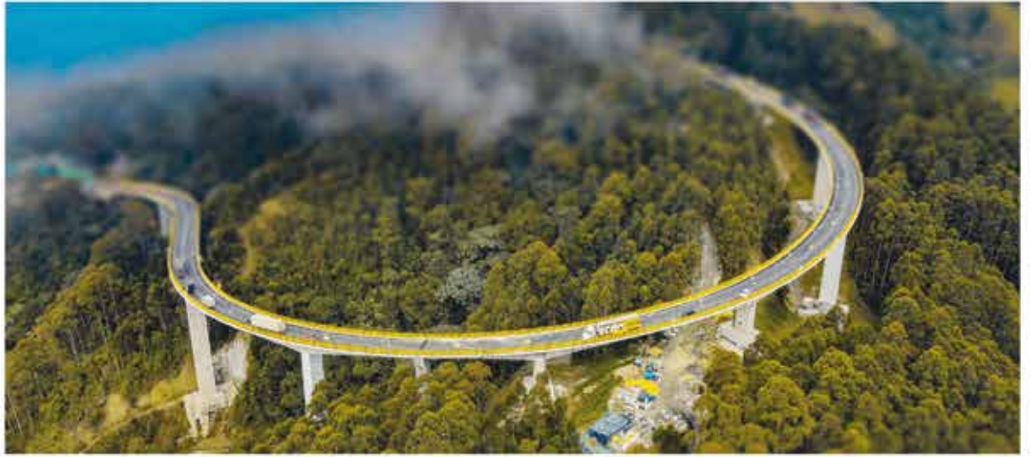
The horseshoe-shaped Yarumo Blanco Viaduct in Colombia significantly reduces travel time from Bogota to the Pacific. In front on the right at the bottom of the short pier, you can see the concrete cube under which the retrofitted isolators are located.
