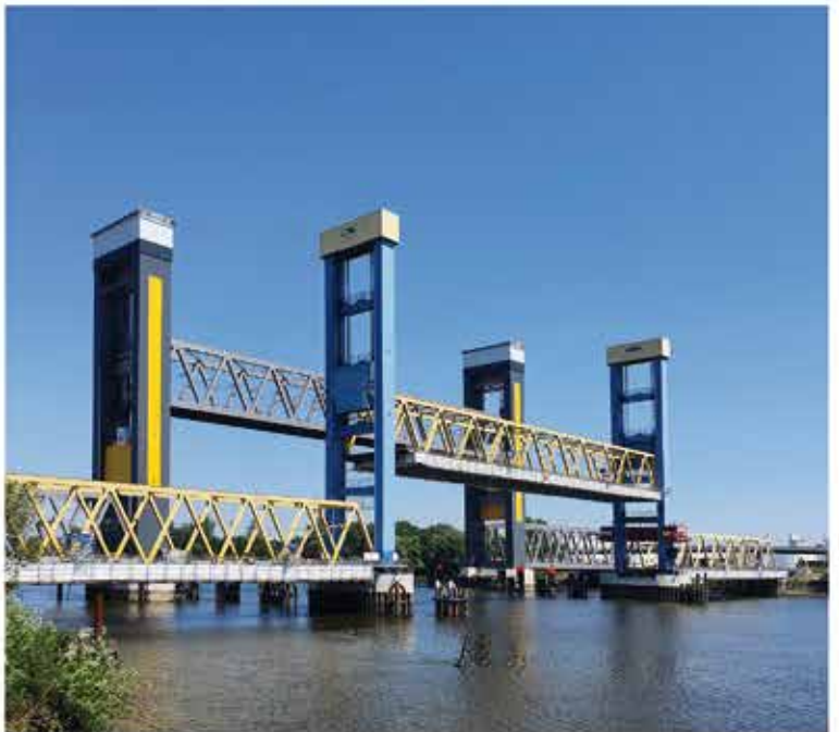
The Kattwyk Bridges in the Port of Hamburg: in the front, the new one for railway traffic, in the back, the one built in 1973, which now only carries road traffic.
