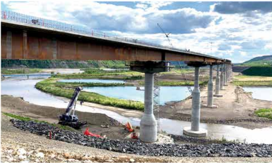
On the left: Halfway River Bridge under construction, May 2021. The tapered piers indicate the future water surface of the reservoir. On the right: Installed bearing with steel girder laid on top.
