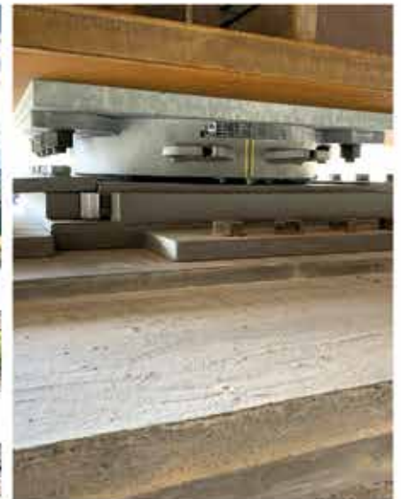
On the left: Halfway River Bridge under construction, May 2021. The tapered piers indicate the future water surface of the reservoir. On the right: Installed bearing with steel girder laid on top.
