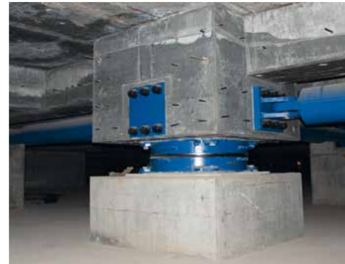
SIP®-A, Djamâ El Djazair Mosque in Algiers
