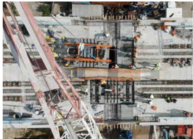
Plan view of Guided Cross-Ties during installation
